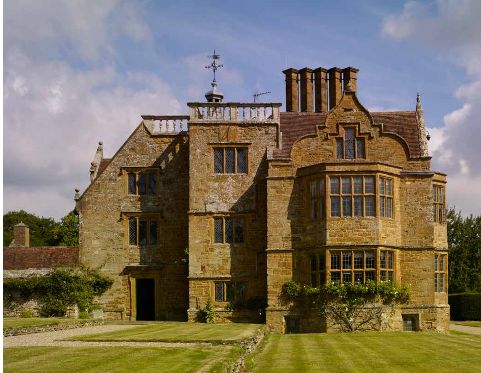
Fig 2: The core of the 17th-century house. The hall gable on the left is connected by a stair turret to John l'Anson's tower, dated 1652
